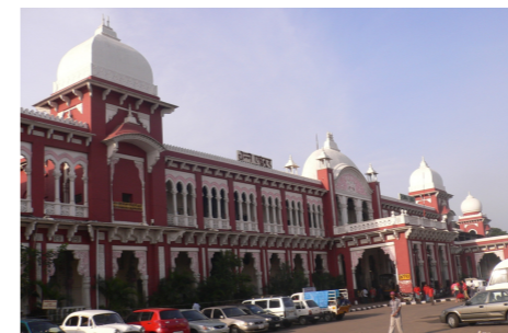
Chennai train station, India
