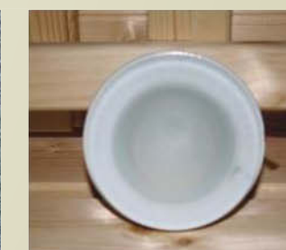
Quartz lamp for steam room lighting
