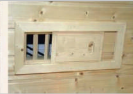
Wooden ventilator sliding grate
